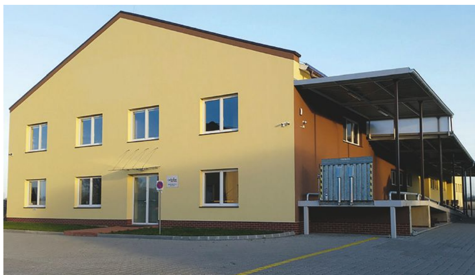
Office and warehouse building of PIROSYSTEM Sp. z o.o. in Wiślina
